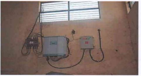
Photo: Solar Control Panel of 30 KWH/Month
